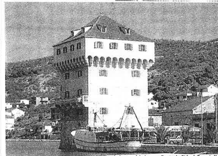
At the bottom of the bay near Trogir: the Bishop's Tower in Murina.
